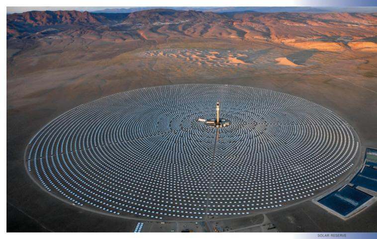
The Crescent Dunes Solar Energy Project near Tonopah is expected to be operational by the end of 2014, and has the capacity to power up to 75,000 homes during peak electricity periods. The project uses 17,500 mirrors to focus the sun's energy, heating salt to molten temperatures. The molten salt is then used to create steam that spins turbines, which creates electricity.
