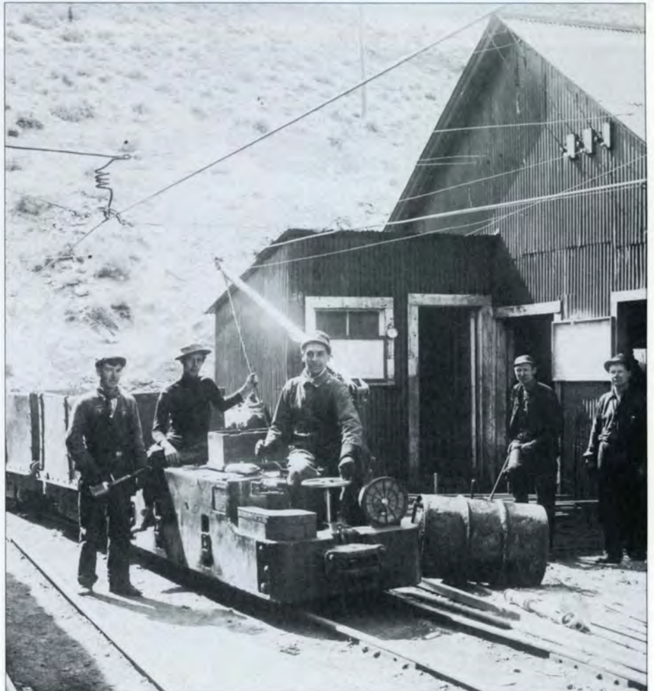
Right: The Mary Mine's entire 13,000-foot tunnel was lit by electricity and had a telephone system linked to all the main workings, according to Hugh A. Shamberger's book, Silver Peak . Thomas Jacques' hand is on the wheel in this photo.
