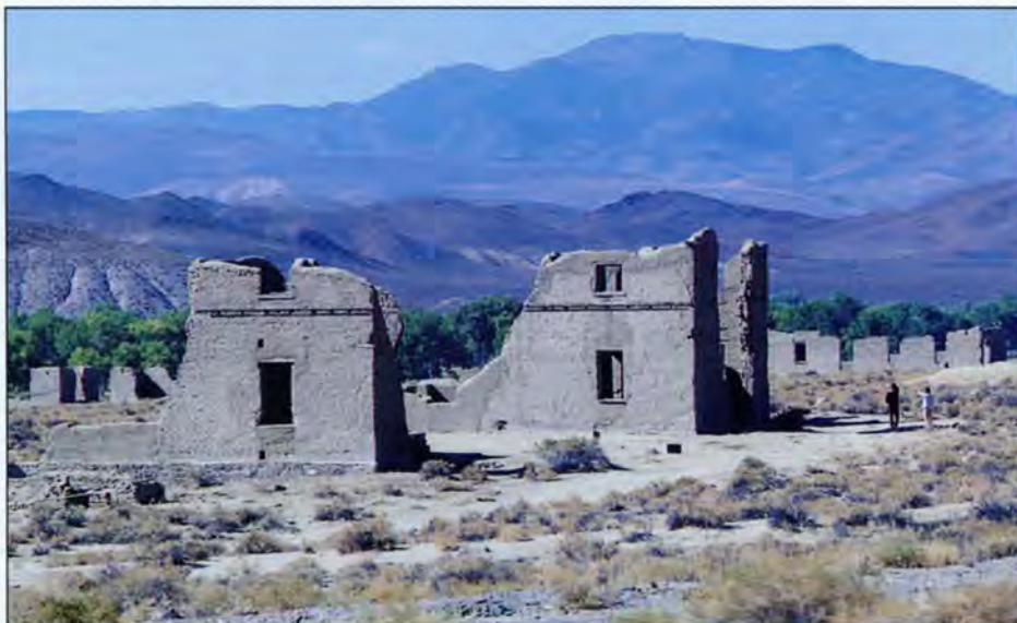
Fort Churchill, built of adobe in 1860, is now a state park on the Carson River
