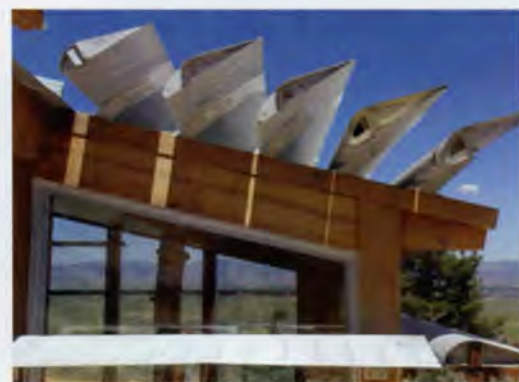
Opposite page: Photovoltaic panels capture solar energy, and a rooftop garden helps insulate the house. Above: Adjustable airplane wing flaps shade tender plants from the intense summer sun.
