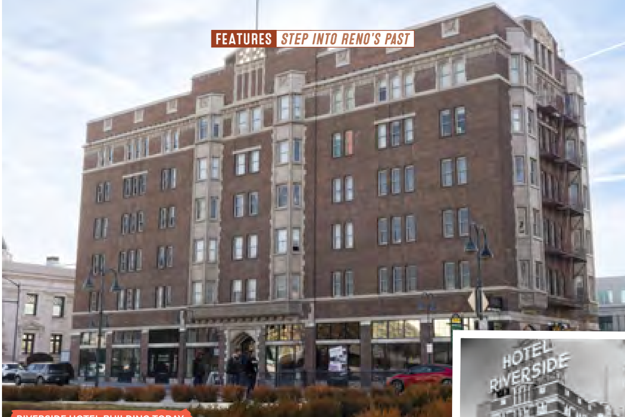
RIVERSIDE HOTEL BUILDING TODAY
