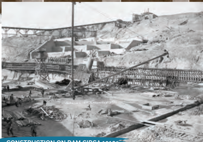
CONSTRUCTION ON DAM CIRCA 1910s
