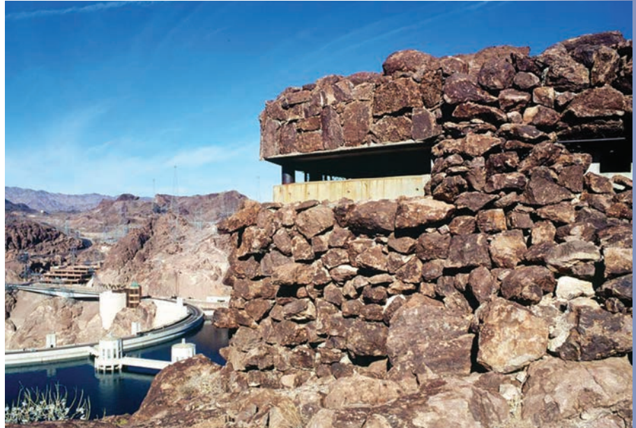
A machine gun pillbox constructed during World War II to protect Hoover Dam. They were constructed of reinforced concrete that was then veneered with native rock found at each emplacement site, blending the bunkers into the craggy cliff walls to avoid detection.
